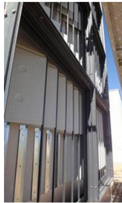
Figure 6. Distribution of PCMs on ventilated facades [58].
